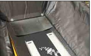
Fig 111 - Tail flashing on top of side flashing
