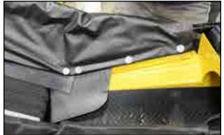
Fig 112 - Transition corner flashing in place
